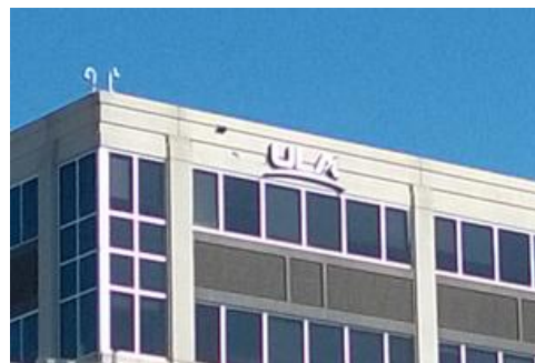
MARK HARDEN | DENVER BUSINESS JOURNAL A ULA office building in Centennial.
